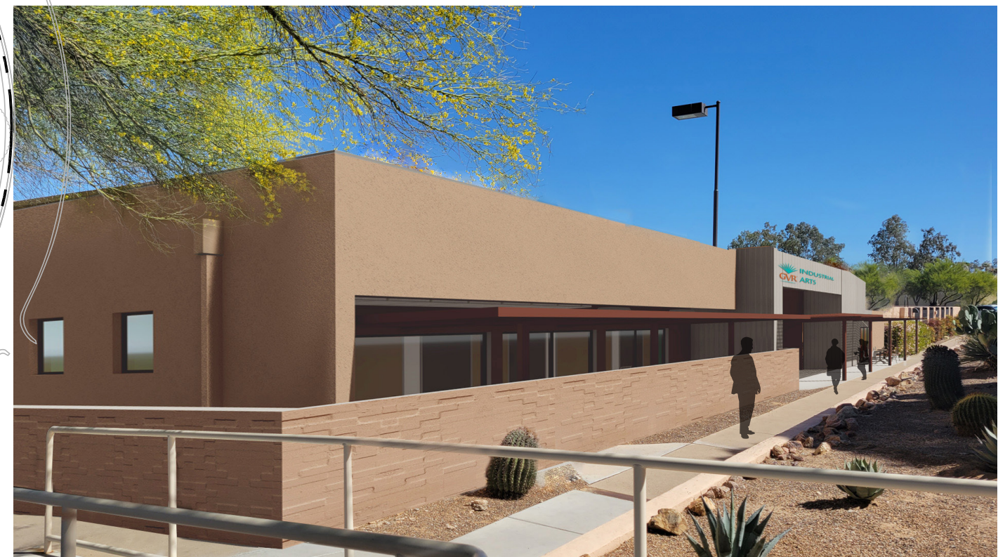
VIEW OF NORTHWEST CORNER
